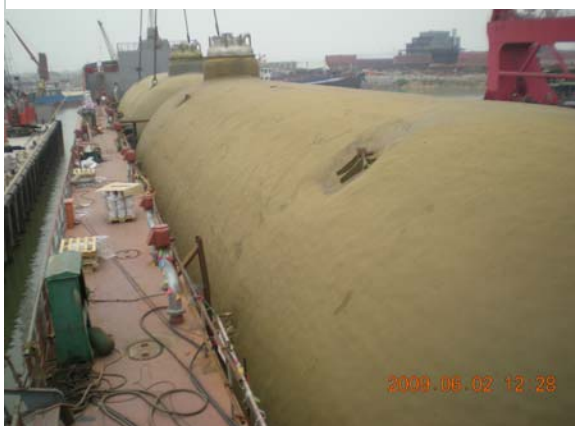
Norgas Innovation – 1 st Multigas vessel is succeeded in Cargo tank installation.
