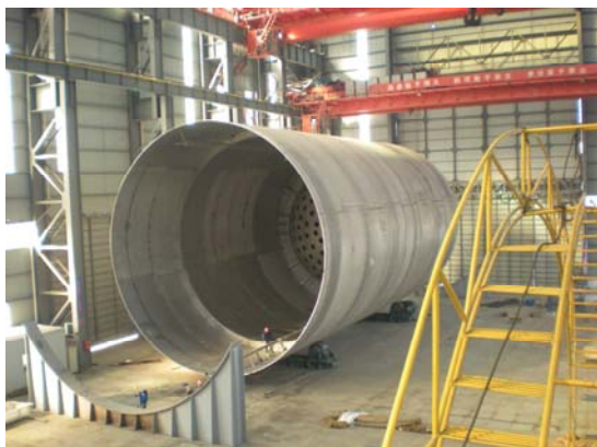
Cargo tank for Norgas Innovation (MG#1) under final construction at Shenghui
