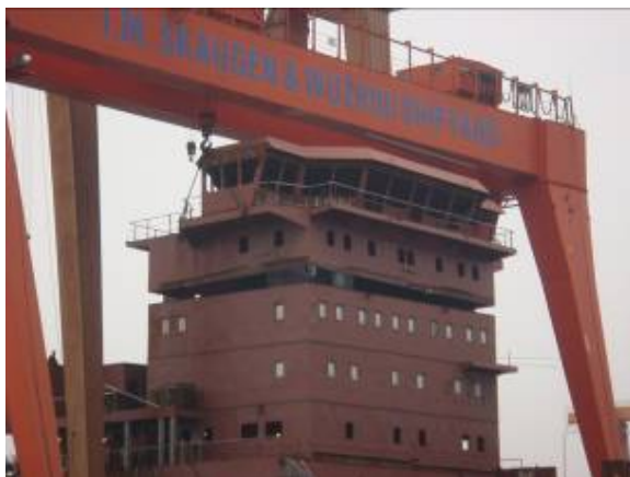
Wheelhouse being lifted onto Multi Gas # 1 at the IM Skaugen Wuzhou Shipyard
